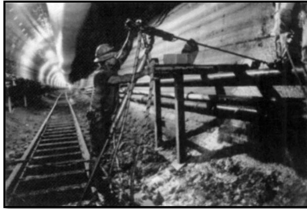
*Figura 63. Taladro Jack leg neumático. Tomado de: Practical guide to grouting of underground structures.*
