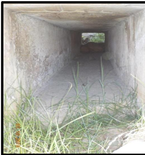
Figura 15 Box Culvert cuenca Soaquira
