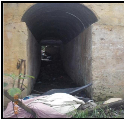
Figura 16 Box Culvert cuenca Soaquira
