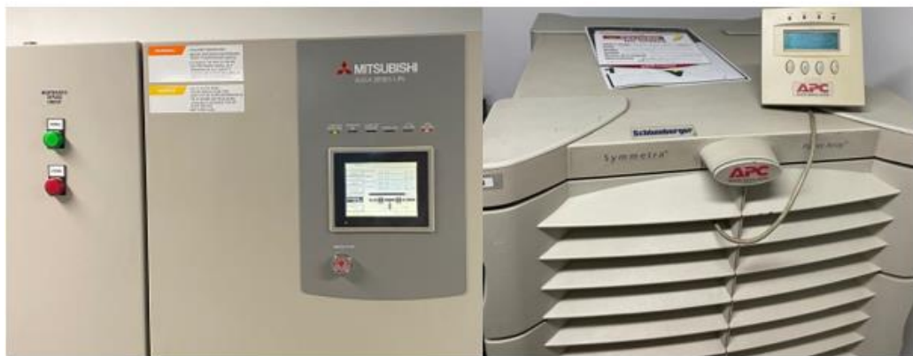
Figura 7: Redundancia de UPS.
