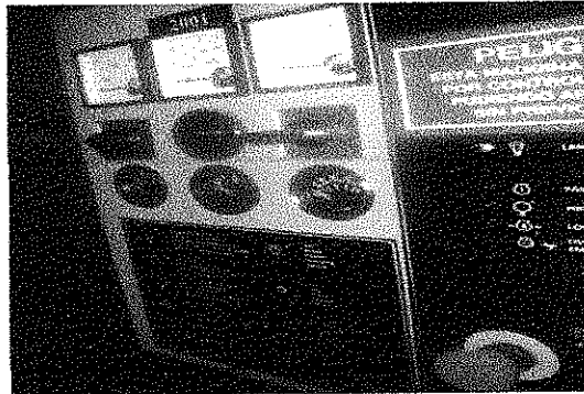
Fig.21 Tablero de control de motor Diesel
