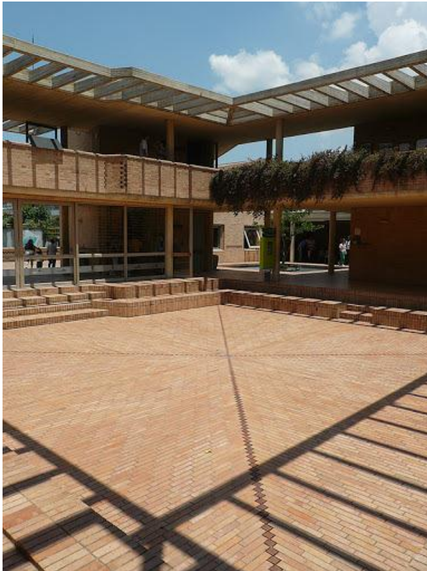
Figura 75. Interior patio central
