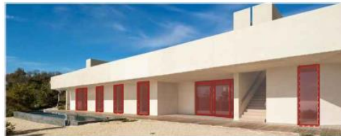
Figura 5. Montauk House, Long Island, USA
