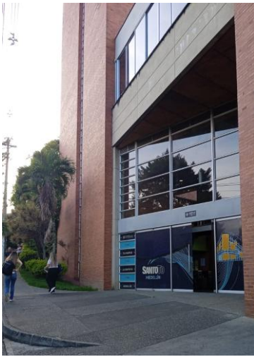
Access ramps, (Building...)
