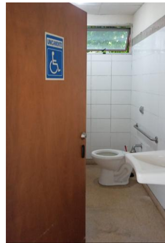
Accessible toilet, (Building...)
