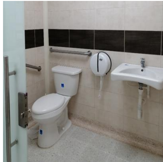
Accessible toilet, (Building...)
