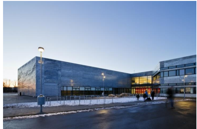
Fig. 29. Acceso al New City School, Frederikshavn, 2012
