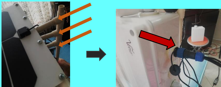
Figure 20. Solar panels removing.
