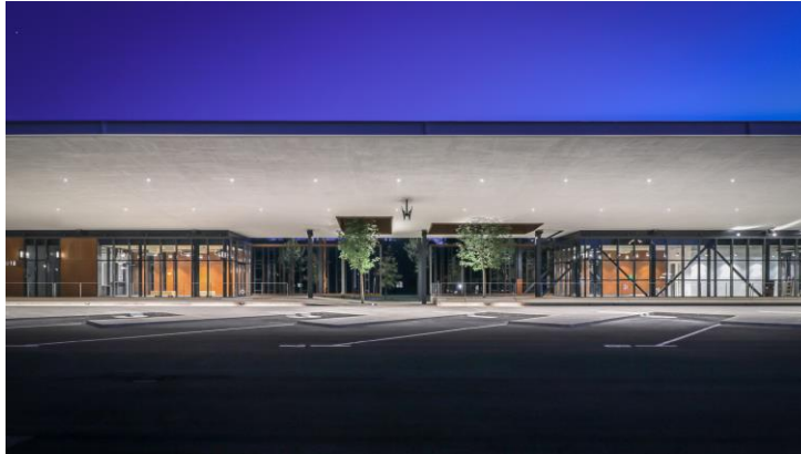
Figura 25 Fachada Terminal Slavonski Brod
