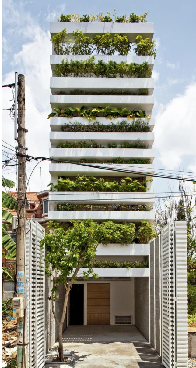
Figura 16. Fachada Stacking Green house
