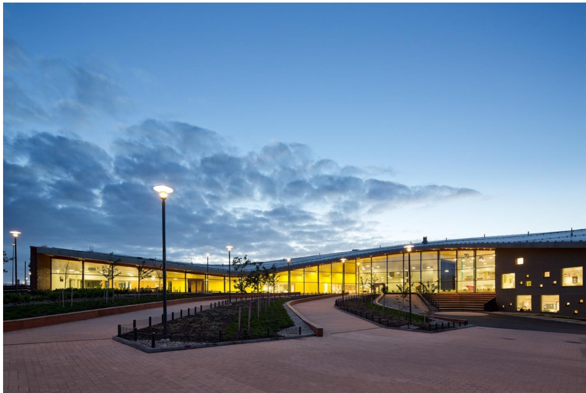
Figura 13. Fachada del Saunalahti School.
