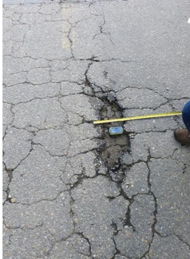
Figura 12.12 Baches (BCH), P68; Sev. A; K0+237.40 Fuente: [22]
