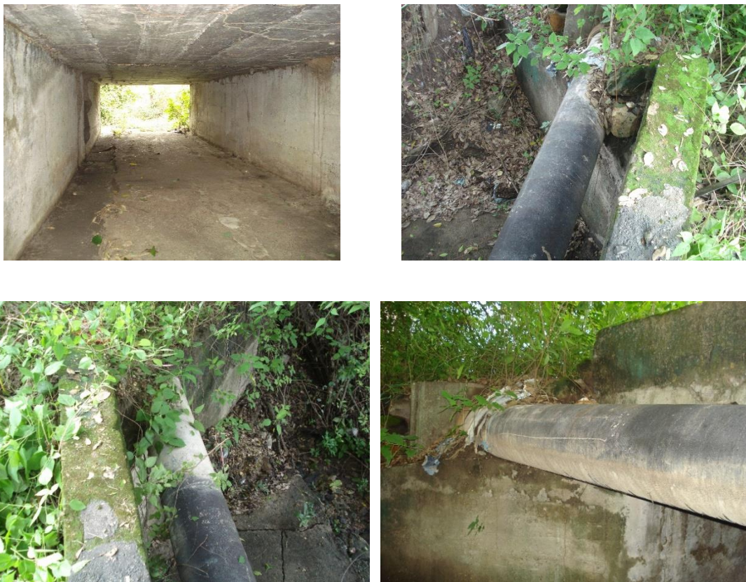
Figura 12 Vista general Box Coulvert K5+629
