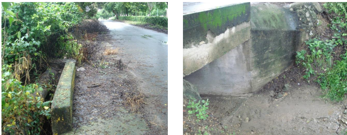
Figura 15 Vista general Box Coulvert K5+105
