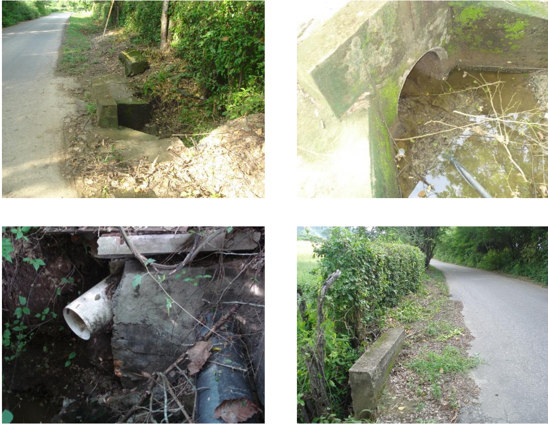
Figura 11 Vista general alcantarilla K5+360
