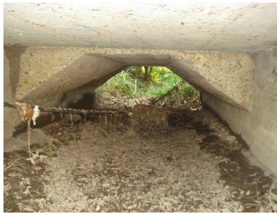
Figura 10 Vista general box Coulvert K5+283
