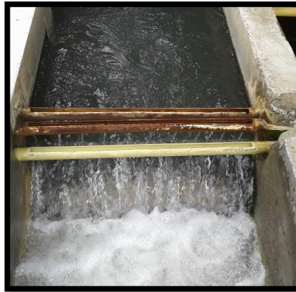
Figura 7: Vertedero rectangular- Pared delgada
