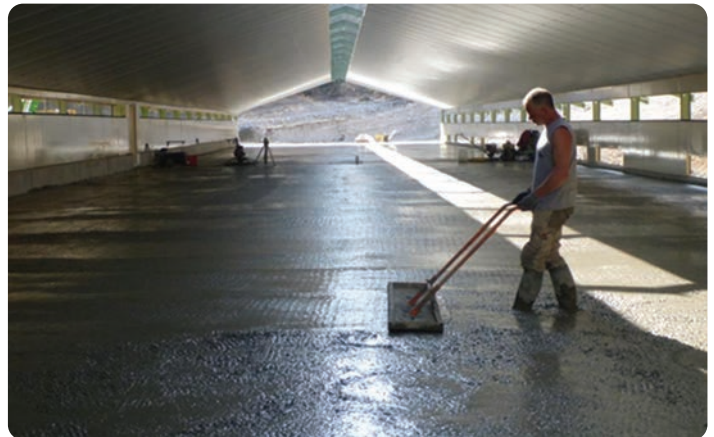
Farm floor – France. 7 kg/m 3 Anti-CRAK® HP 67/36, C 30/37
