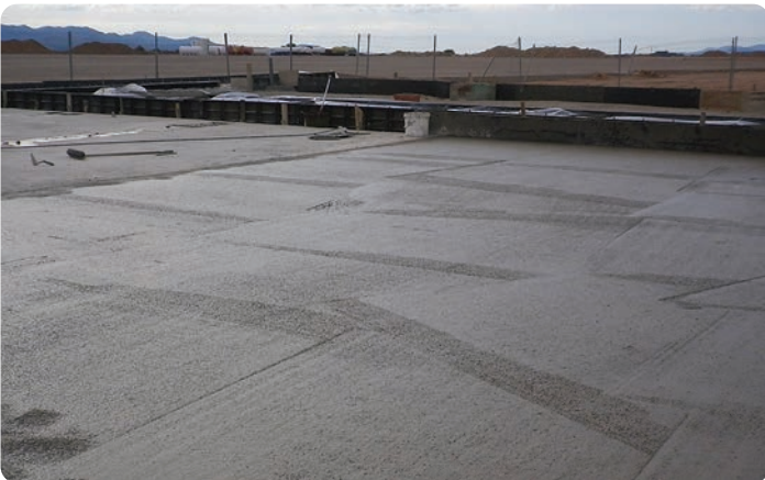
Airport pavement – Aeródromo T-35, AVIALSA, Spain. 5 kg/m 3 Anti-CRAK® HP 67/36, C 30/37.
