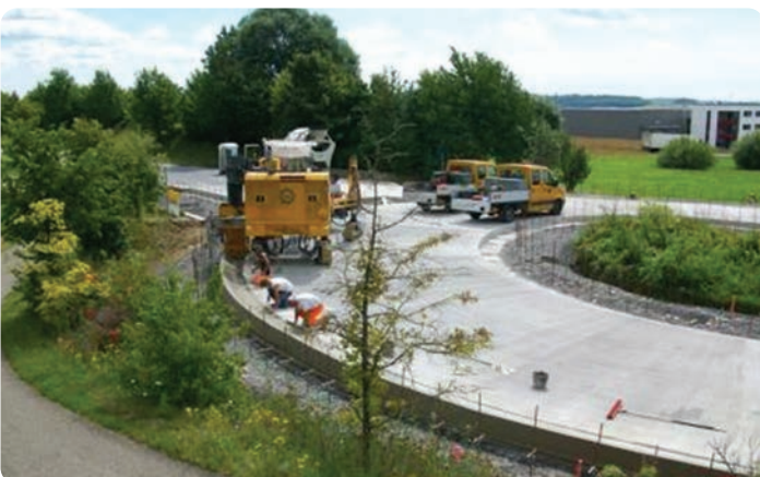
Roundabout – Road K 1060/1013, Germany. 10 kg/m 3 Anti-CRAK® HP 67/36, C 30/37
