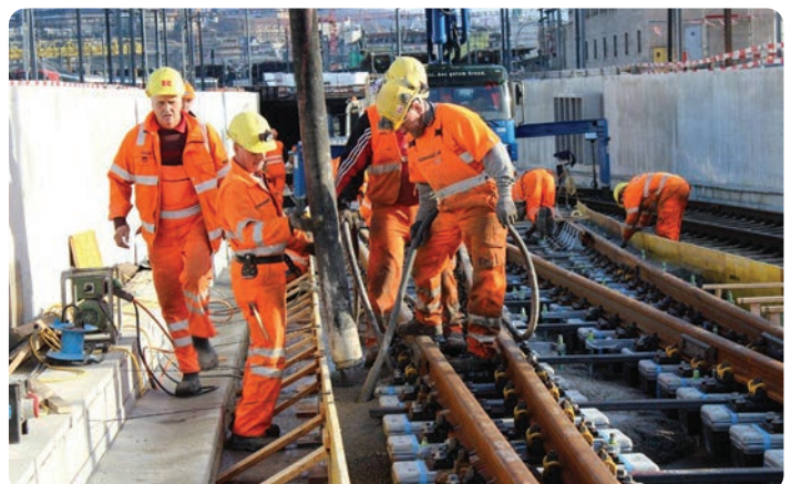
Railway base – Zurich Diameter Line, Switzerland. 8 kg/m 3 Anti-CRAK® HP 67/36, C 25/30
