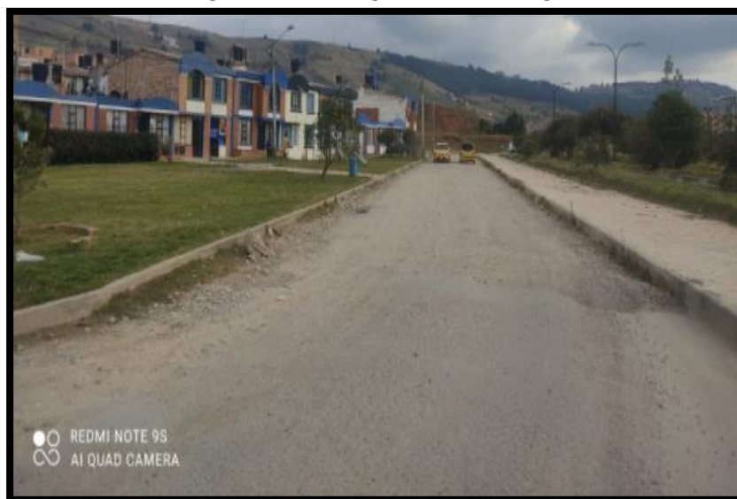
Figura 72. Tramo 17 A. diagonal 4 a diagonal 3e - diagonal 4c.
