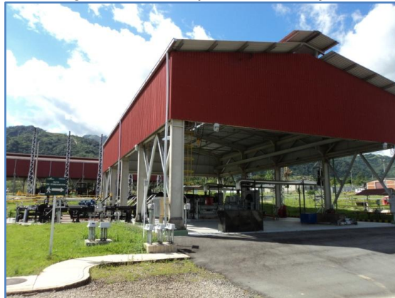
Fig. 8. Casa-maquina Monterrey II.
